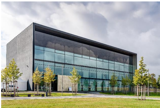
Image 1: The facade of the Casting Technology Laboratory of Fraunhofer IGCV | Copyright: Fraunhofer IGCV / Andreas Heddergott
